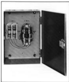
FIGURE 5-30. TYPICAL AUTOMATIC SHORELINE TRANSFER SWITCH
