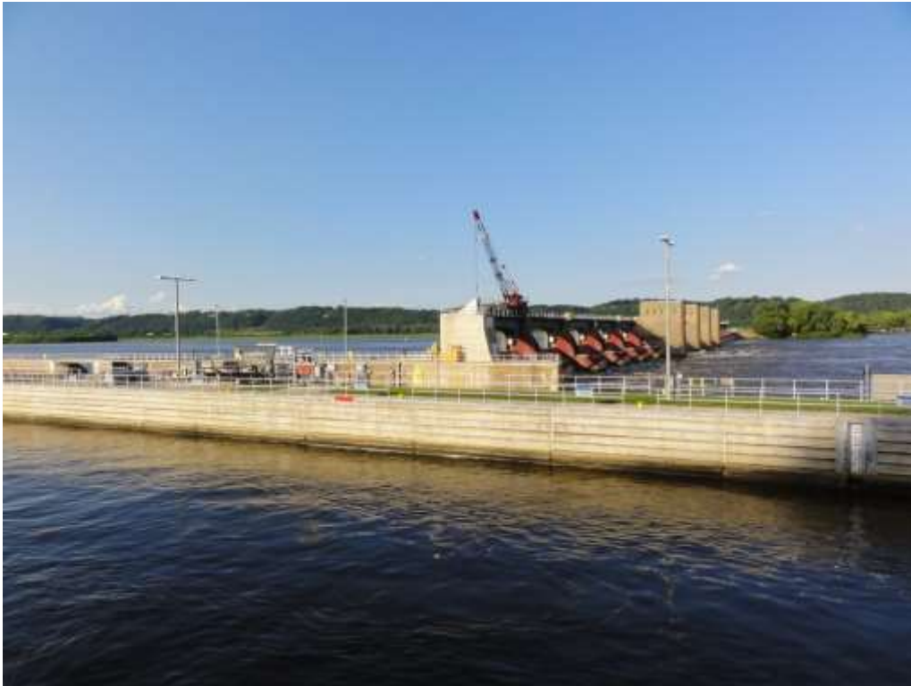
Lock & Dam at Dubuque
